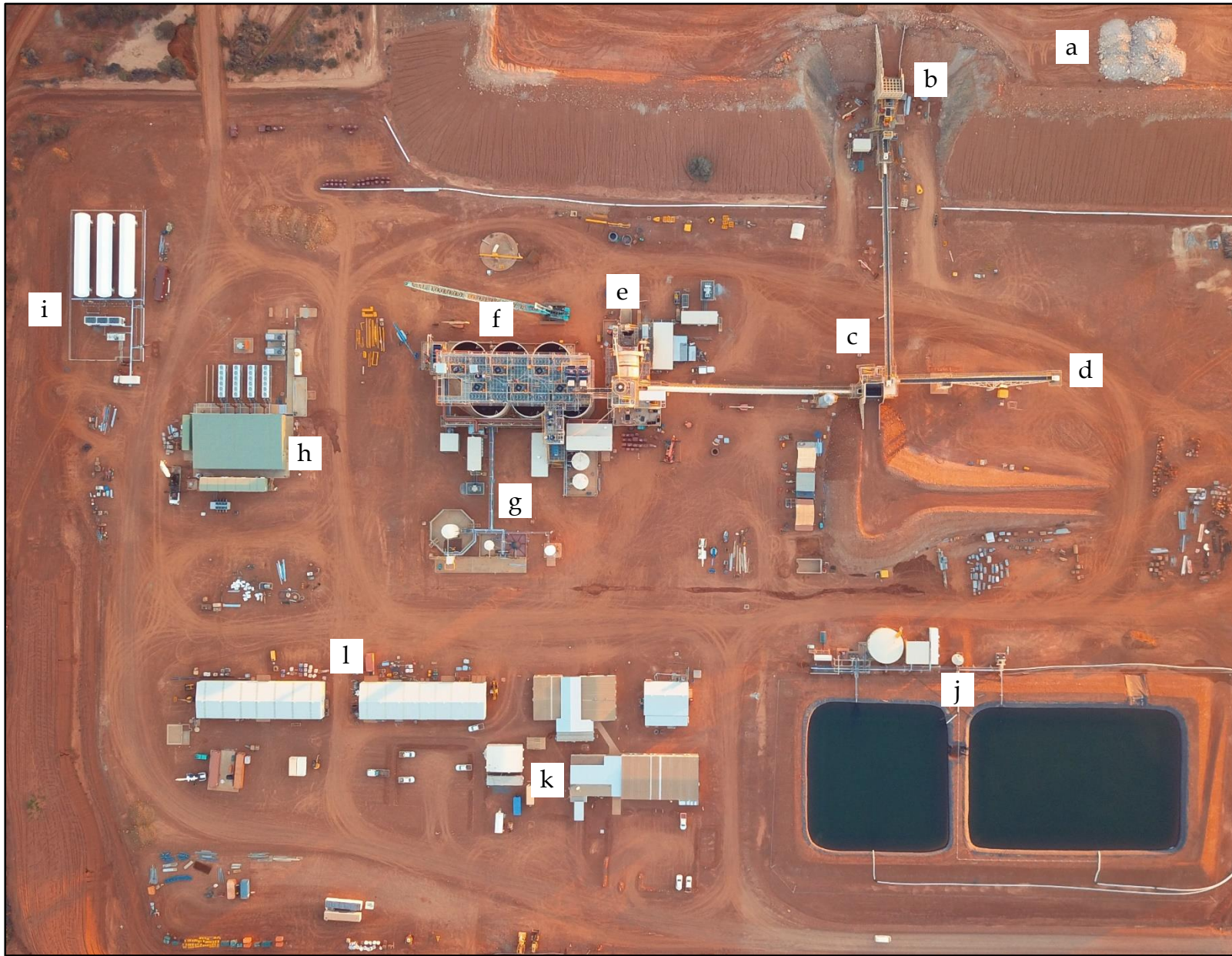
Photo 2: Dalgarranga Process Plant Site Overview
