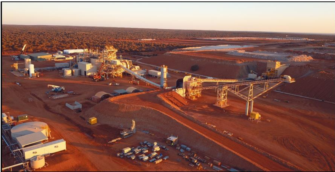
Dry commissioning of the process plant is underway
