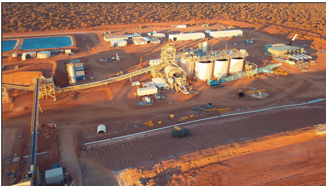
Photo 1: Dalgaranga Plant Site Construction Progress
