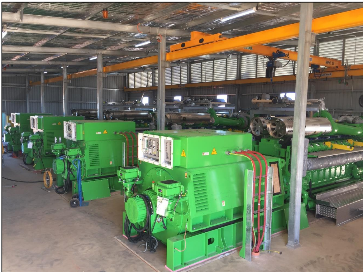
Photo 10: Installation of the Jenbacher Gas Fired Generators Underway
