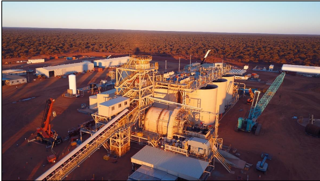
Photo 3: SAG Mill Installation – Nearing Completion
