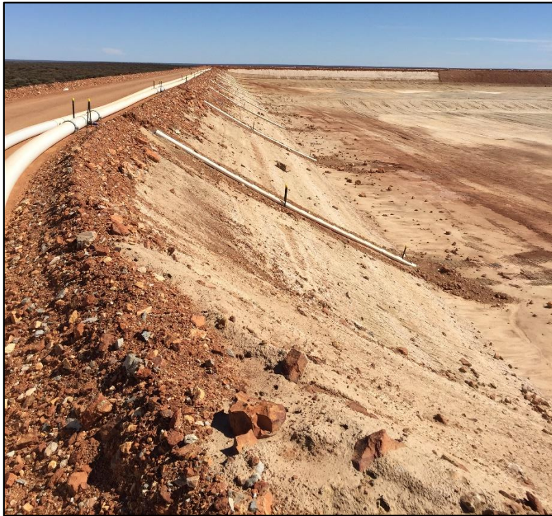
Photo 13: Dalgaranga Tailings Storage Facility Ready for Use
