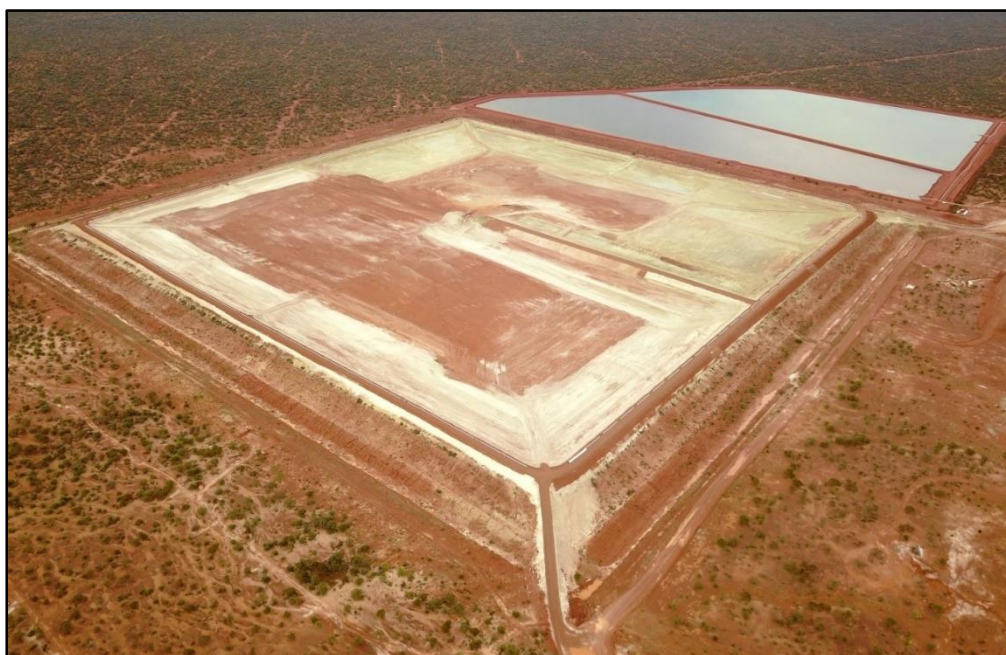
Photo 12: Dalgaranga Tailings Storage Facility Ready for Use (foreground) and Evaporation Ponds In Use (background)
