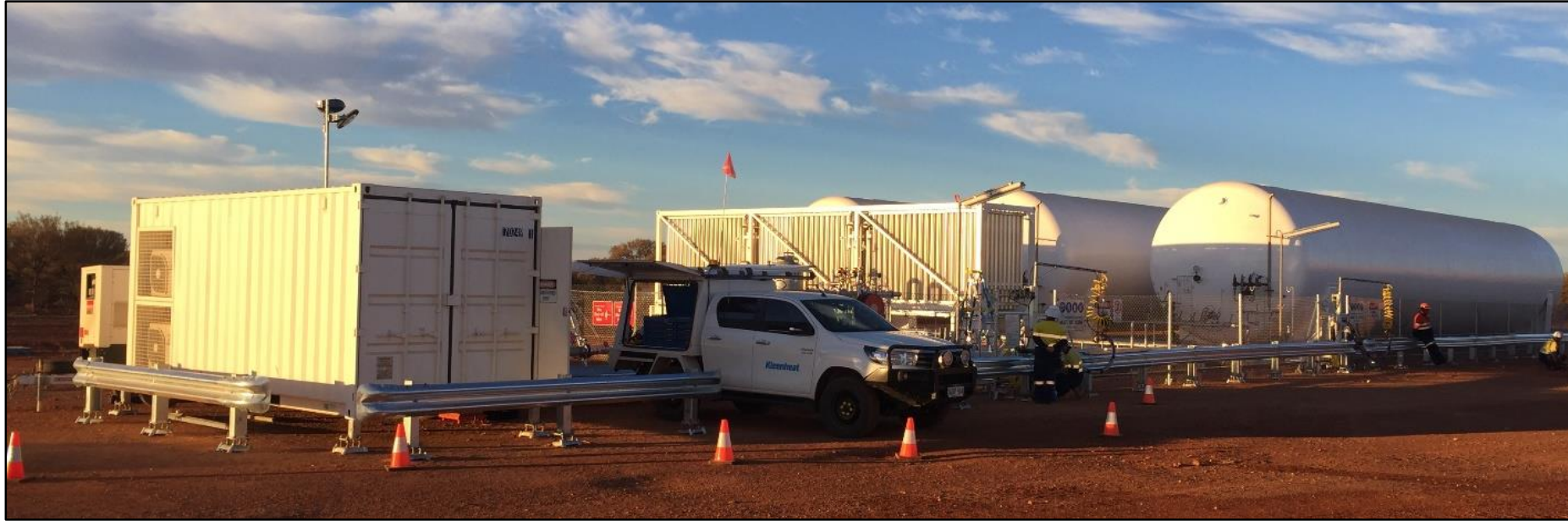
LNG Storage Facility – Commissioning Underway
