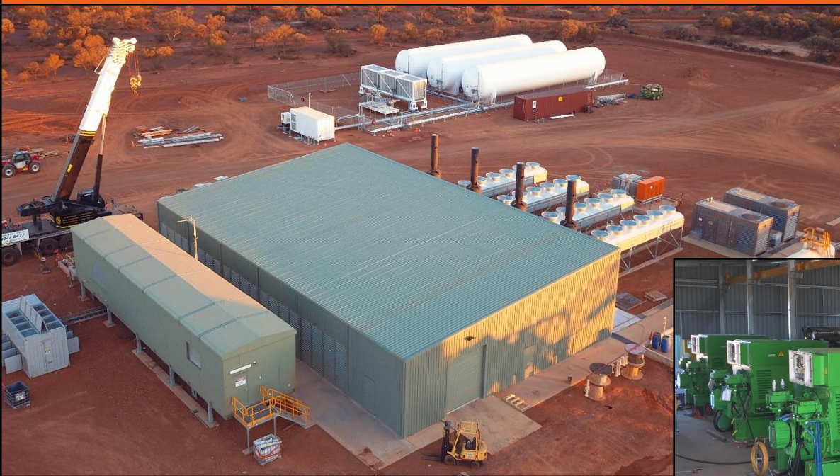
Power Station Construction – Well Advanced
