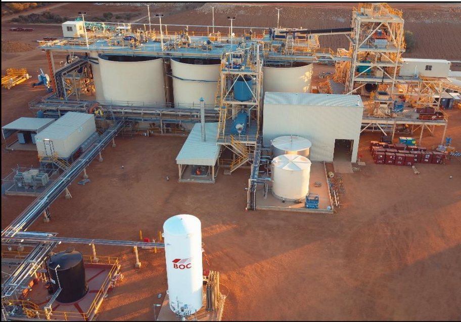
Top of CIL Tank Steelwork, Cyclone Tower and Reagent Storage
