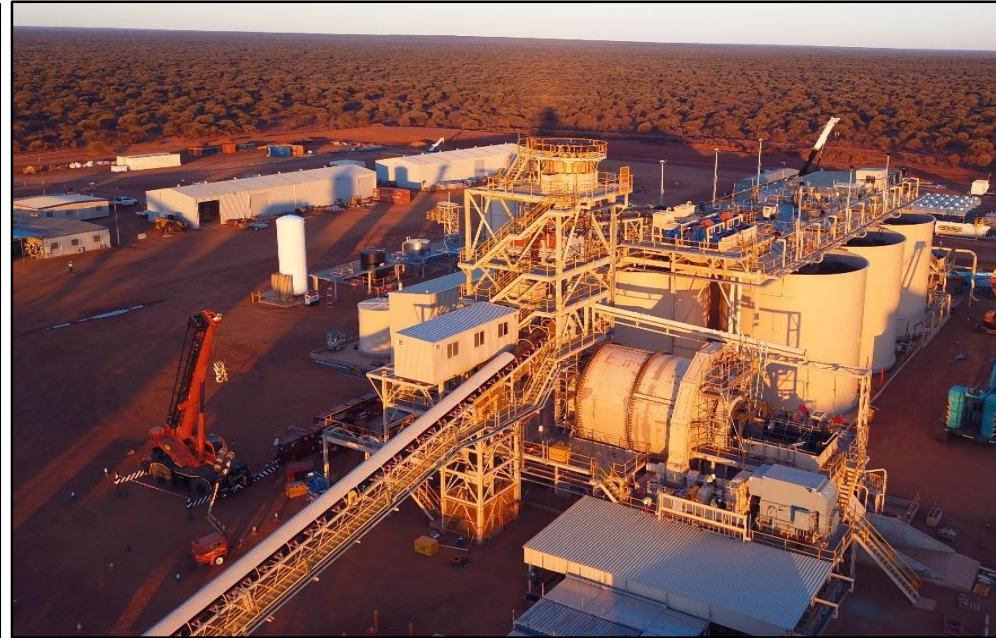
SAG Mill Installation – Well Advanced
