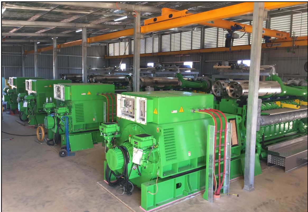
Photo 10: Installation of the Jenbacher Gas Fired Generators Underway
