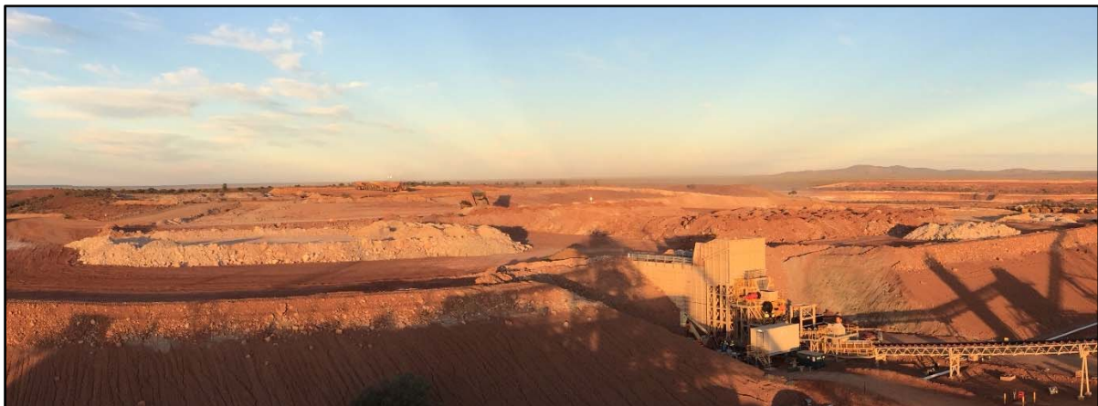
Photo 8: ROM Ore Stockpile being developed ahead of Processing
