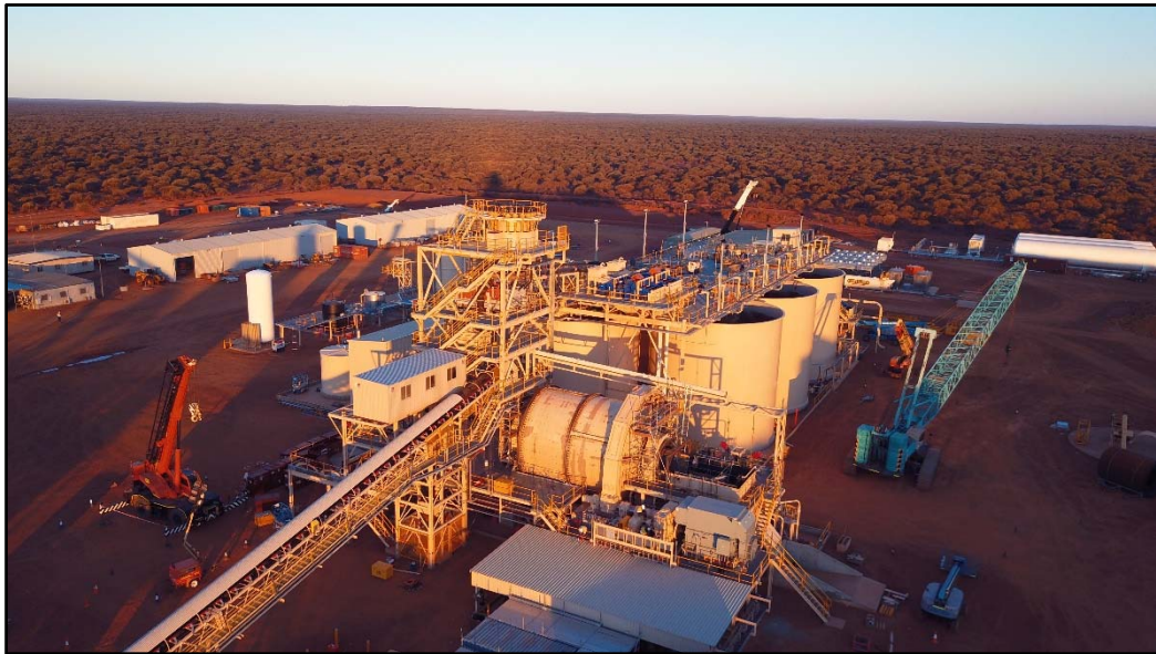
Photo 3: SAG Mill Installation – Progressing Well
