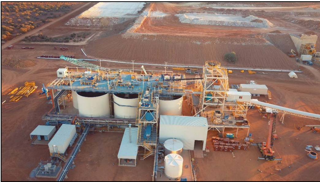
Photo 4: Cyclone Tower Construction Complete and Installation of Mechanical Equipment – Nearing Completion
