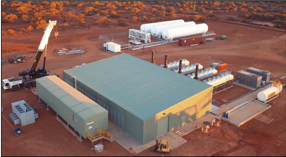
Photo 9: Zenith's Engine Hall and HV Switchroom & EVOL's LNG Storage Facility
