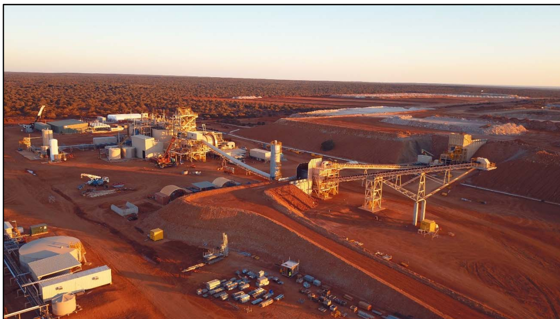
Photo 1: Dalgaranga Plant Site Construction Progress
