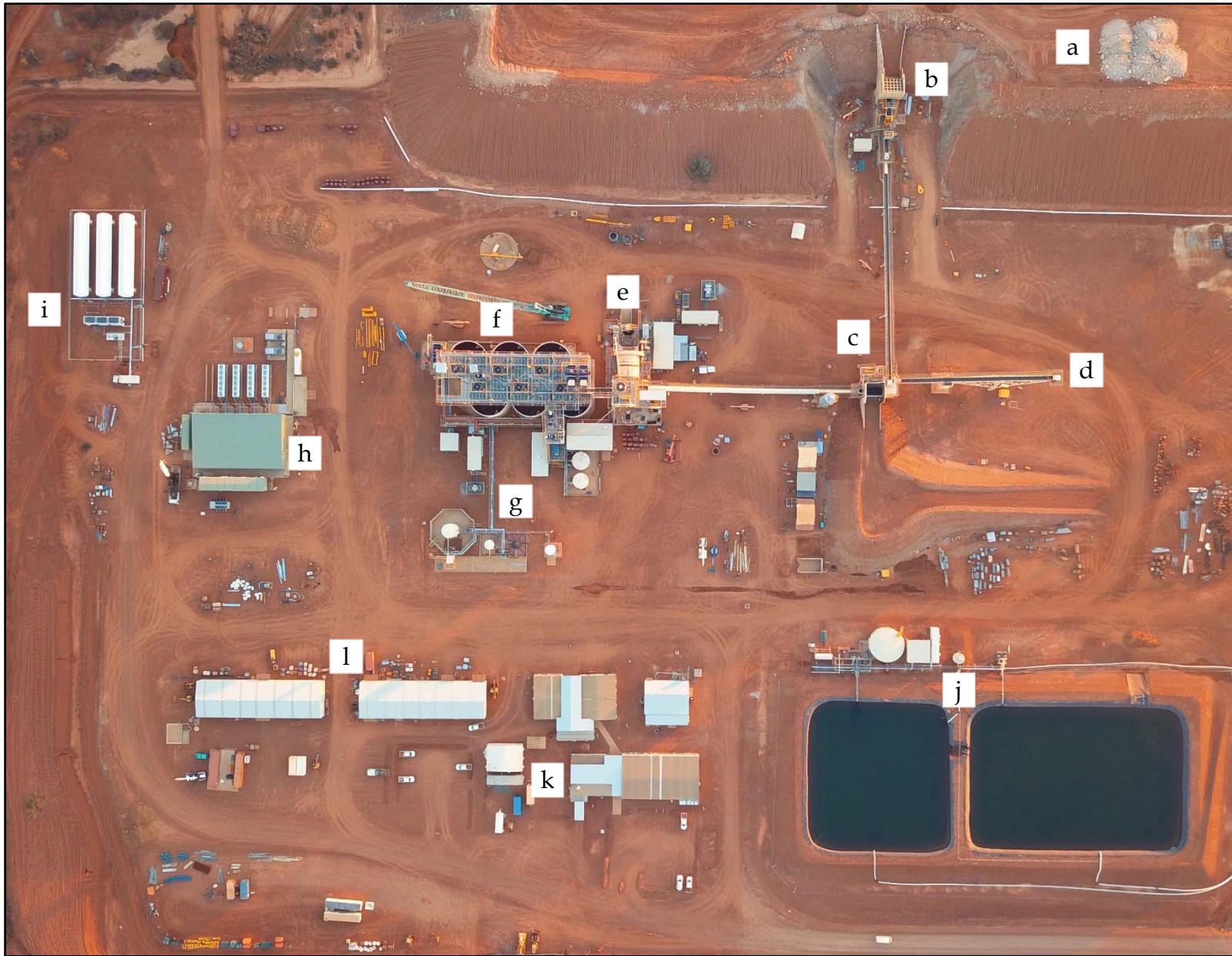
Photo 2: Dalgara Process Plant Site Overview
