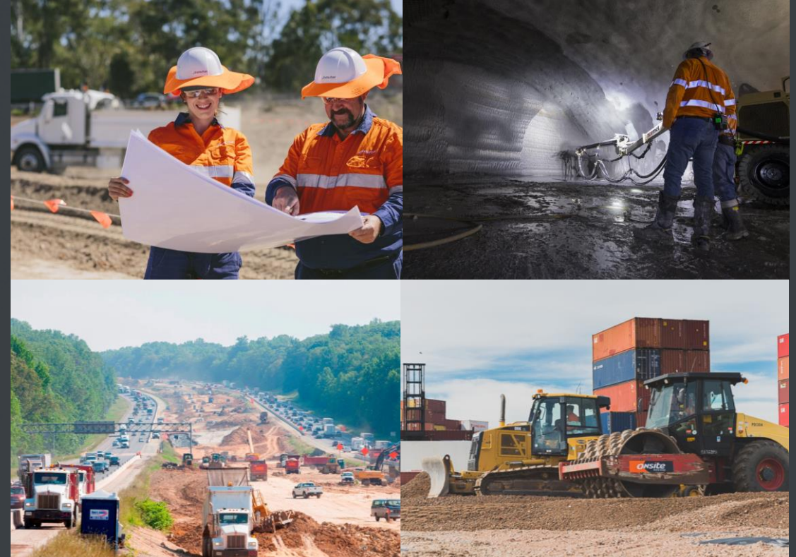
LEP, NorthConnex, 395 Express Lanes and West Gate Tunnel projects all submitted under proposals frameworks
