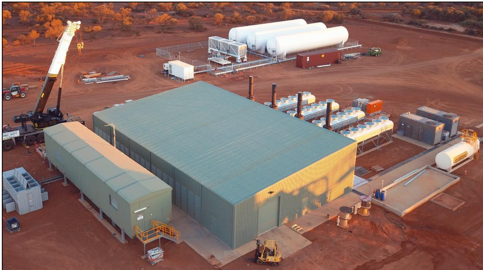
Power Station & LNG Storage facility – Operational
