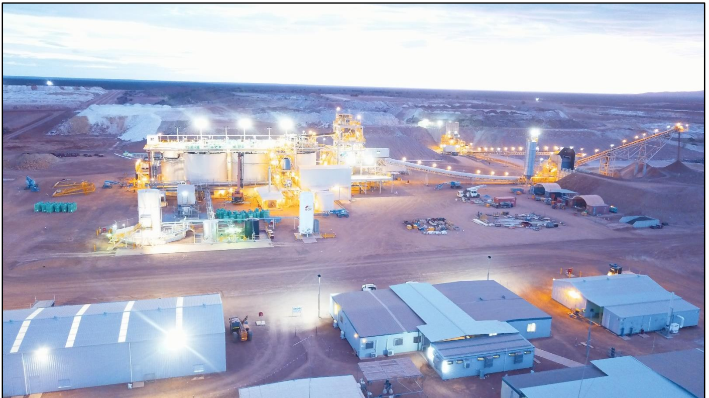
Dalgaranga Gold Project 2.5Mtpa Processing Facility
