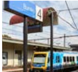
Burnley Train Station Burnley
