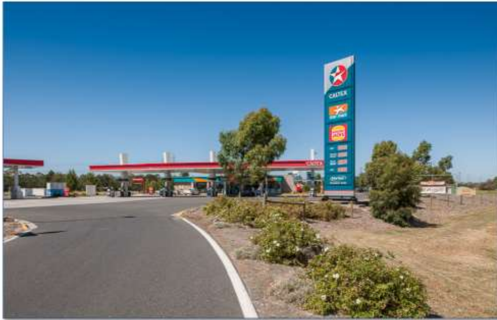
Caltex Longwarry Eastbound (view from service land off the Princes Highway)
