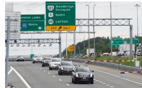
Automated vehicles operating on the reversible 95 Express Lanes
