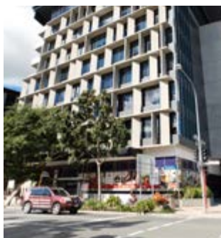
SW1 Complex, South Brisbane, QLD (5 properties)
