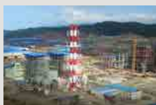
1.2GW power station &amp; coal plant
