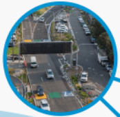
Ground access work
