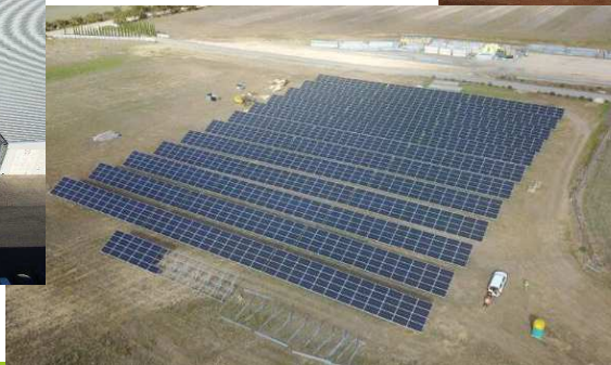
First stage of new solar farm installation
