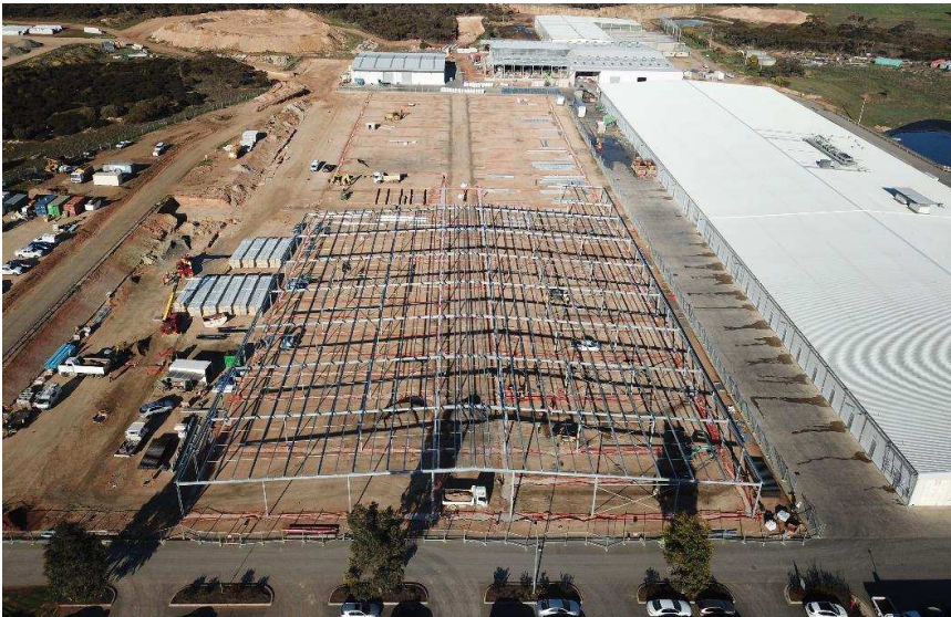
Monarto farm expansion in progress
