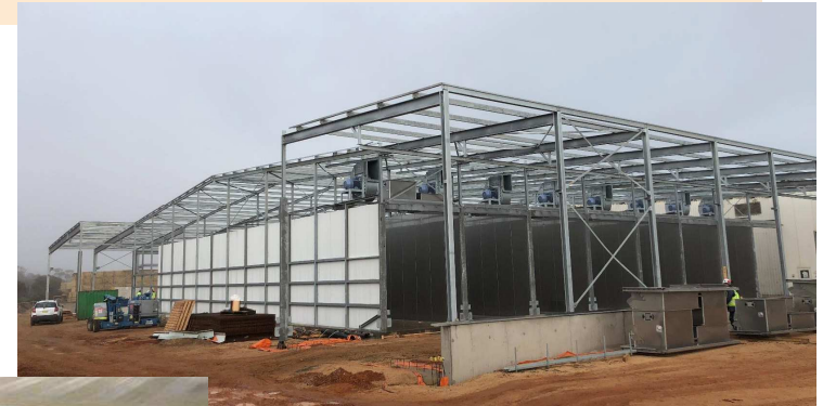
Compost bunkers under construction
