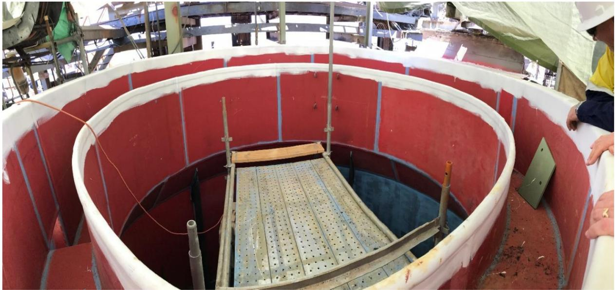
*New rubber lining in the flotation cells*
