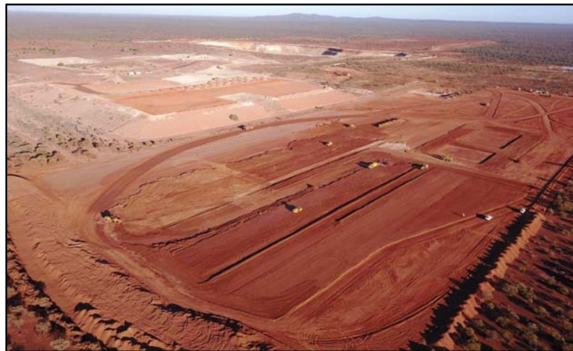
Photograph 1: Commencement of Civil Earthworks August 2017
