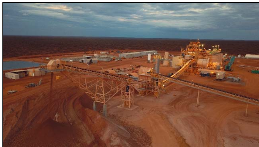
Photograph 2: Process Plant Commissioning May 2018
