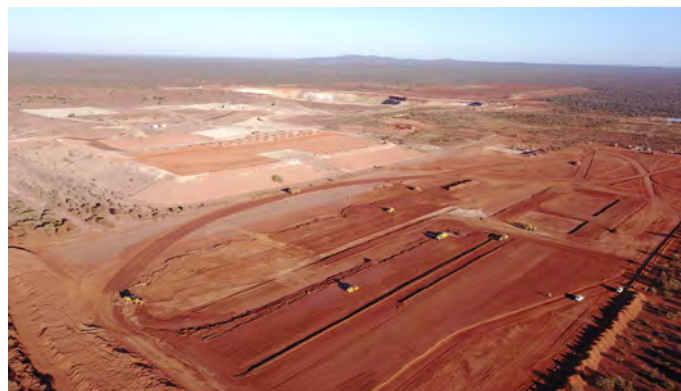
Photograph 1: Commencement of civil earthworks August 2017
