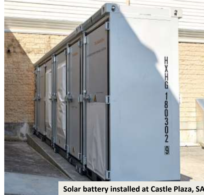
Solar panels at Castle Plaza, SA
