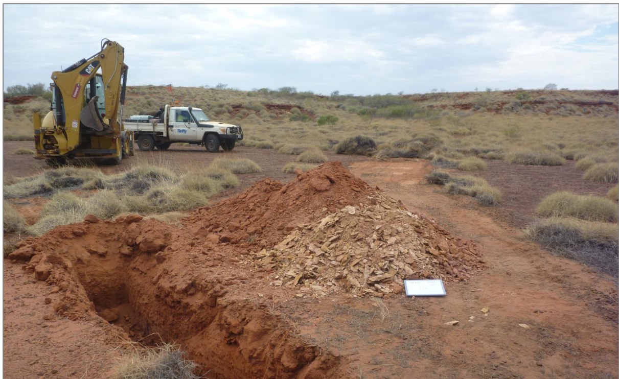
Figure 4. Haul Road Test Pit in Progress
