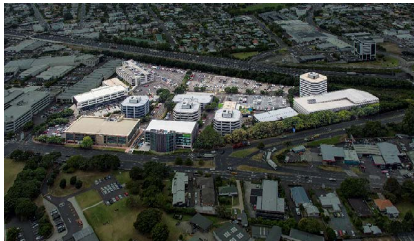
Central Park Centre, Greenlane, Auckland
