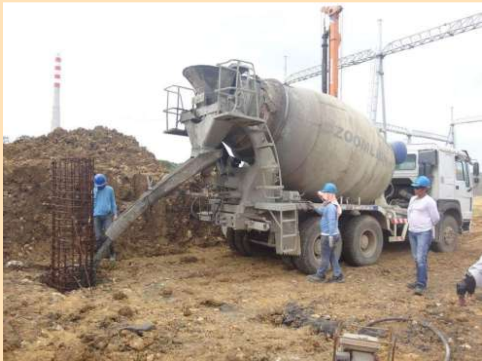
Concreting of Tower 1 Foundations
