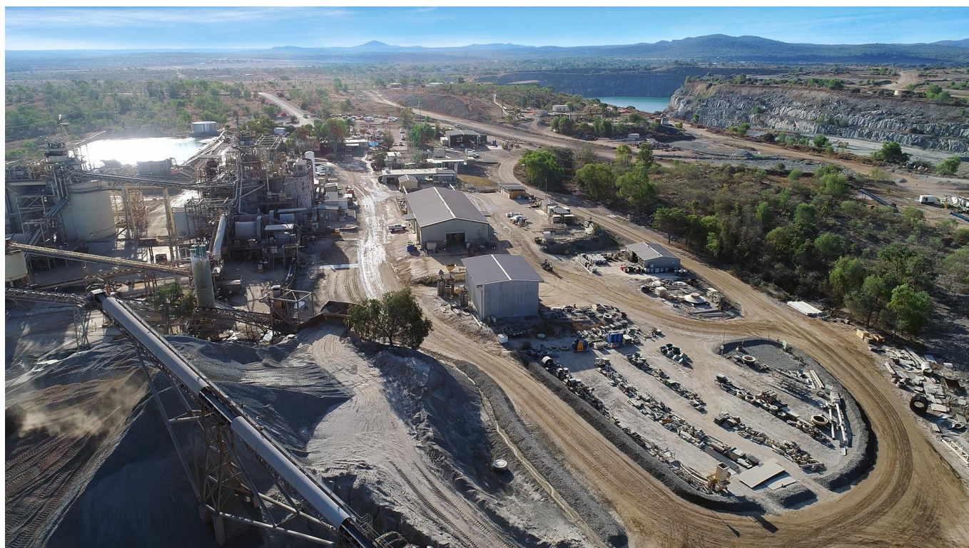
Figure 1: The Nolans Processing Plant and Sarsfield open pit
