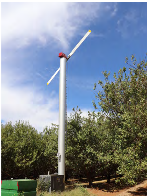
Figure 13: Frost fan installed on Moorral orchard
