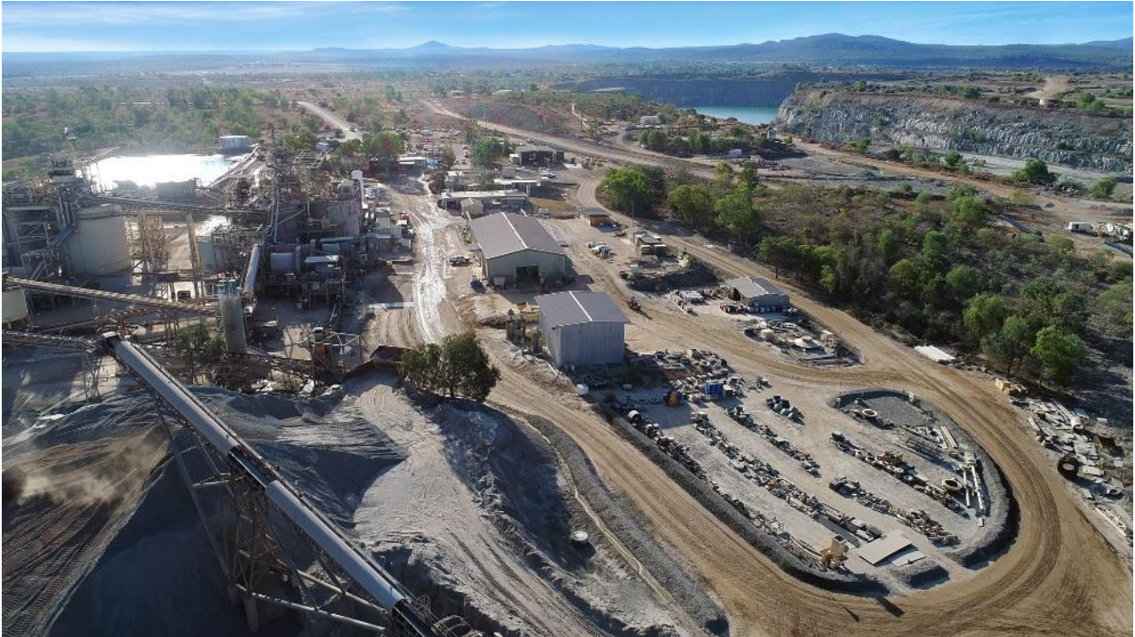
Figure 11: Nolans Processing Plant and Sarsfield Open Pit
