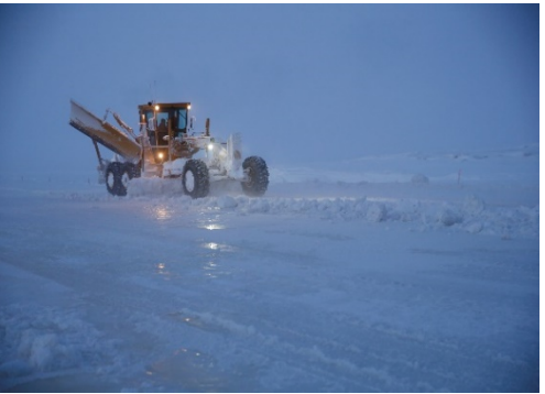
Ice road construction
