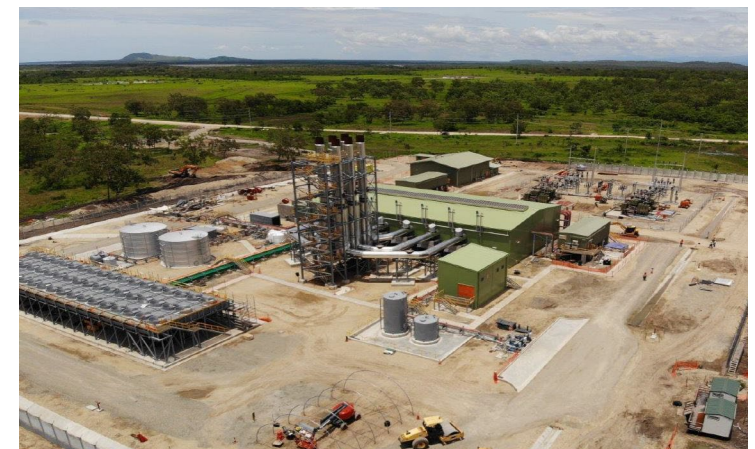
58MW gas fired power station, located adjacent to PNG LNG plant site January 2019
