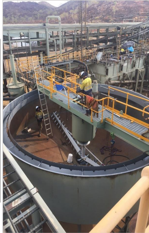
Refurbishment of tails thickener
