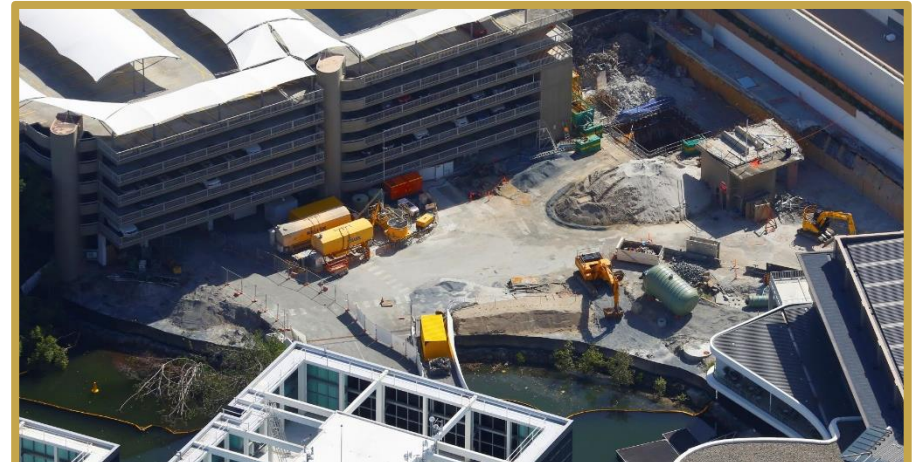
DORSETT HOTEL AND RESIDENCES CONSTRUCTION UNDERWAY
