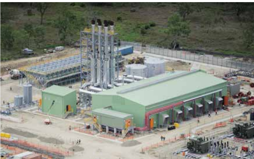
58 MW gas fired power station expected to supply approximately 75% of Port Moresby’s electricity needs.
