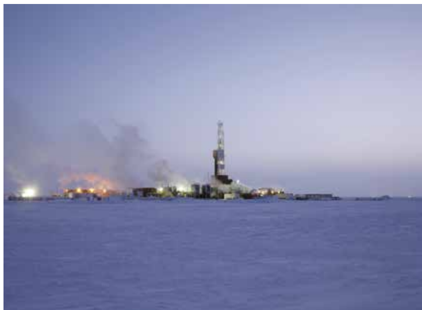
Pikka B well, located on the Alaska North Slope.
