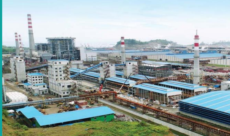
2GW Coal Fired Power Station
