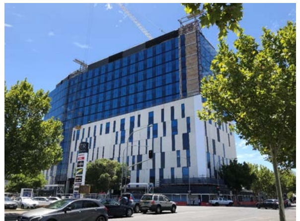
Calvary Adelaide Hospital – under construction.
