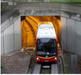
Obahn City Access Project, SA $160 million Project completed
