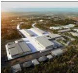
Tindal Air Base R8000, NT $450 million Project in progress
