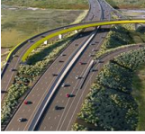
Northern Connector, SA $885 million Project in progress
