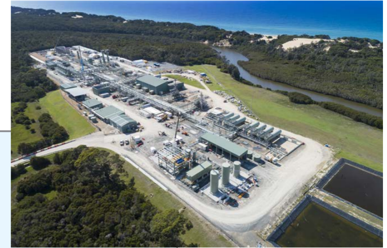
Orbost Gas Plant
