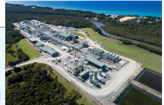
Orbost Gas Plant
