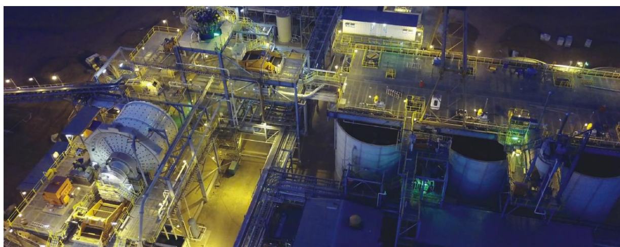
Figure 3: Mako Gold Mine Processing Plant
