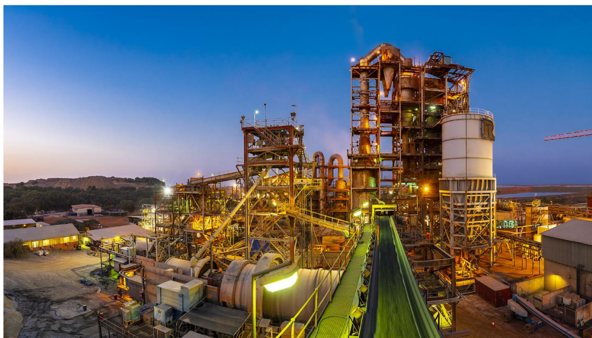
Syama Processing Plant
