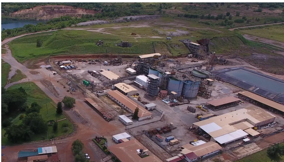
Bibiani Processing Plant and Administration
