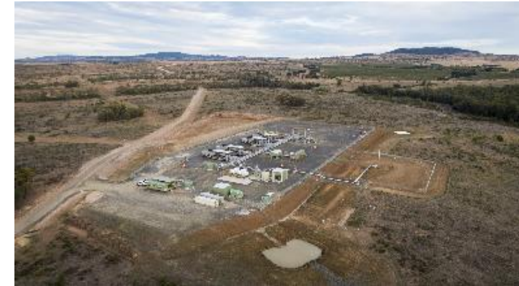
Roma North gas compressor station; 16 TJ/day (~6 PJ/year) initial capacity, expandable to 48 TJ/day (~18 PJ/year)
