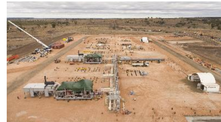
Project Atlas gas compressor station; 40 TJ/day, including 8 TJ/day installed redundant capacity (~15 PJ/year) initial capacity, expandable to 48 TJ/day (~18 PJ/year)
