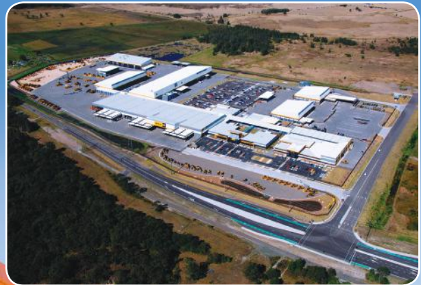
WesTrac Newcastle, aerial view
