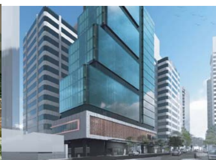
Victoria Avenue, Chatswood NSW
