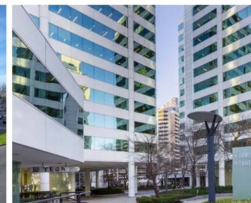
Victoria Avenue, Chatswood
