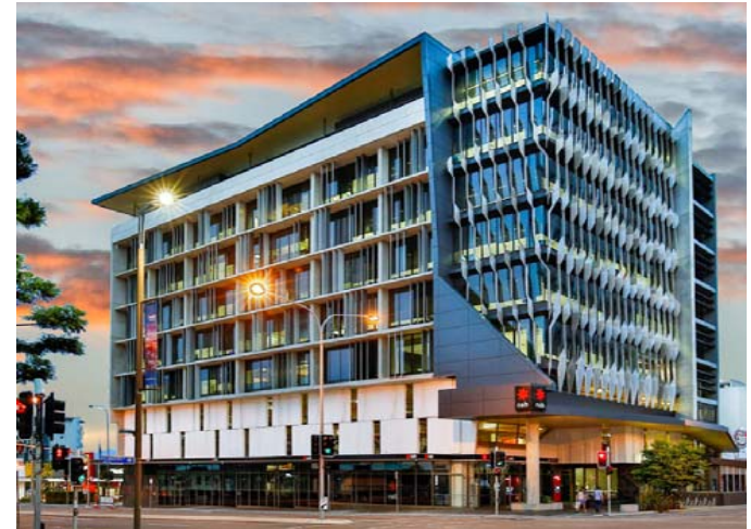
420 Flinders Street, Townsville
