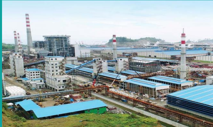
2GW Coal Fired Power Station
