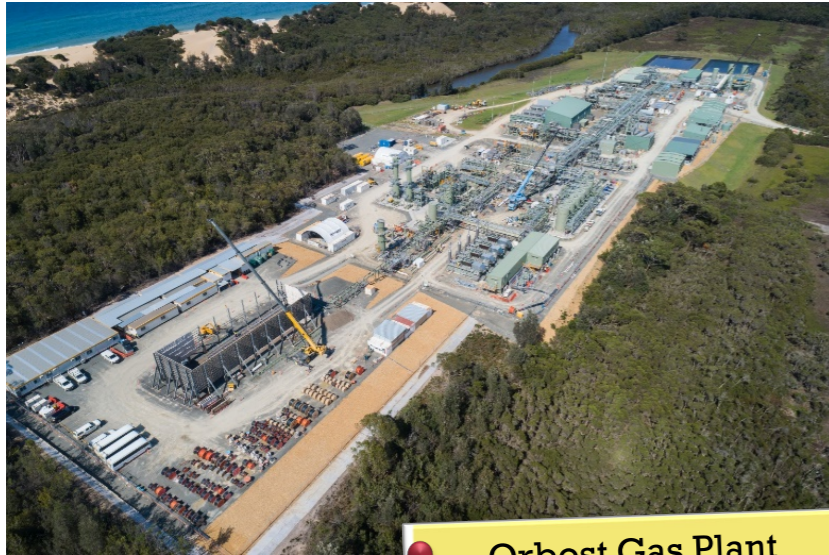
Orbest Gas Plant
