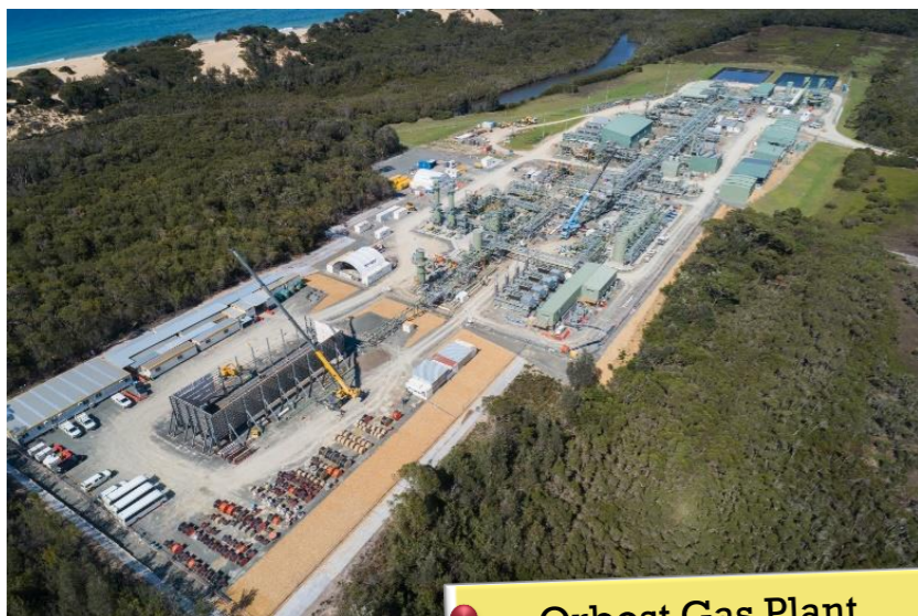
Orbest Gas Plant
