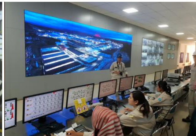
RKEF Control Room
