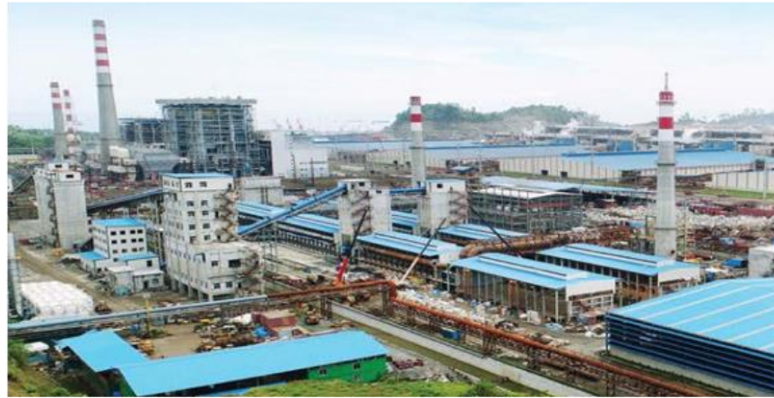
Coal Fired Power Station
