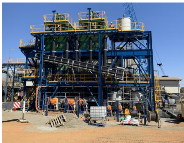
Zinc Flotation Area Construction
