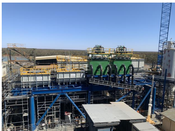
Lead Flotation Area Construction
