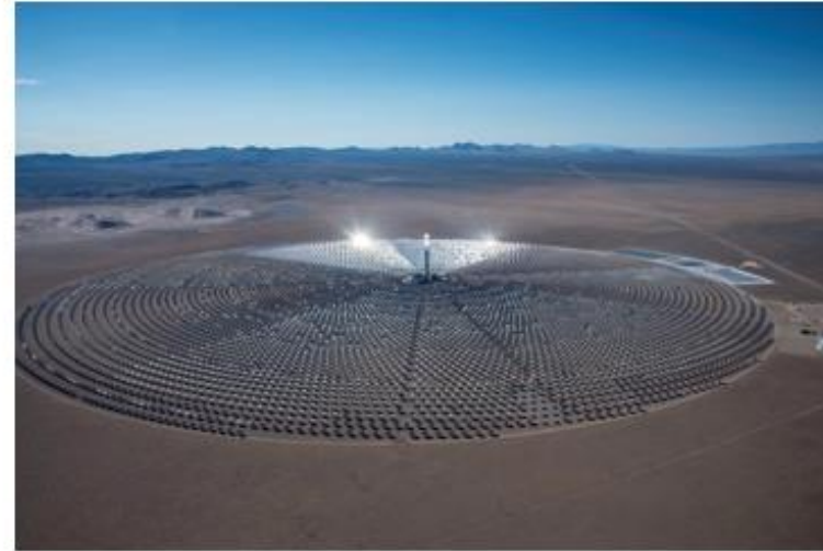
Concentrated Solar Power
