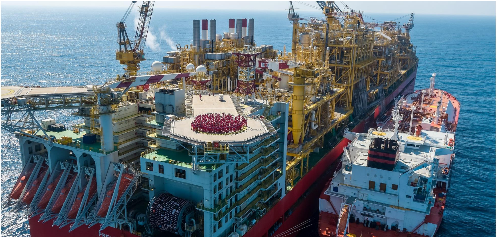
Shell's Prelude Floating Liquefied Natural Gas Facility in Western Australia.
