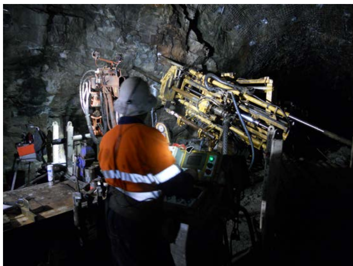
Figure 1 - Underground RC Drilling on 11340 North Section
