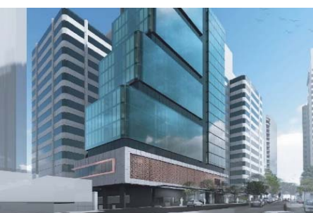
Victoria Avenue, Chatswood NSW
