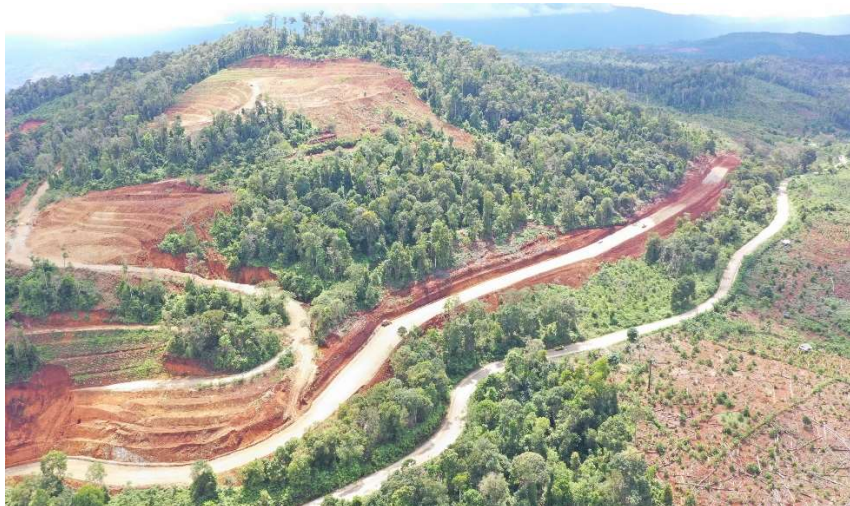
Haul road to Central pit completed
