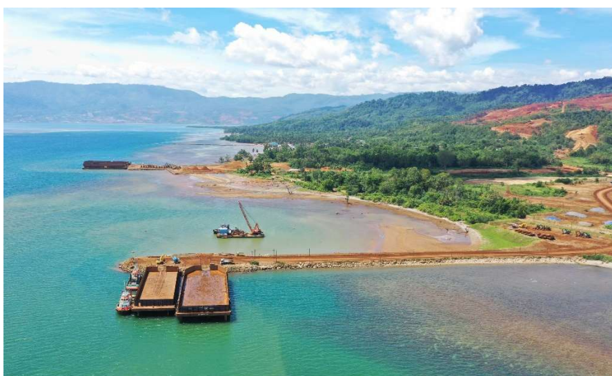
Jetty works underway
