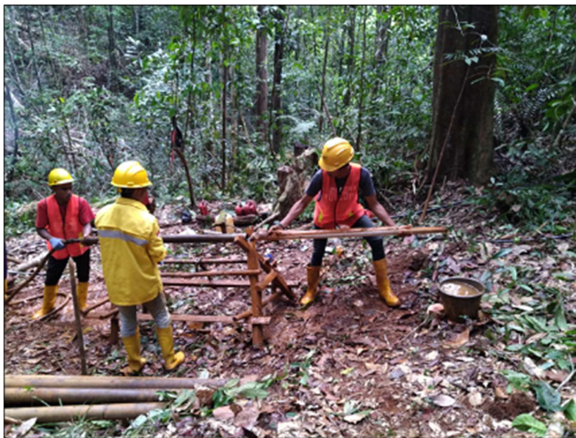
Clearance work in Central pit areas.
