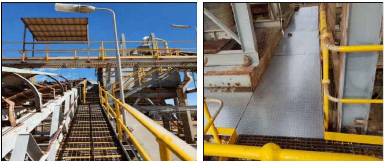
Figure 1 – Black Swan processing facility safety works program – example of completed works
