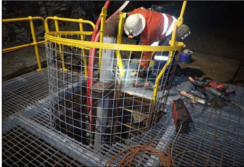
Figure 2 - Silver Swan escapeway ladder refurbishment program – example of completed works
