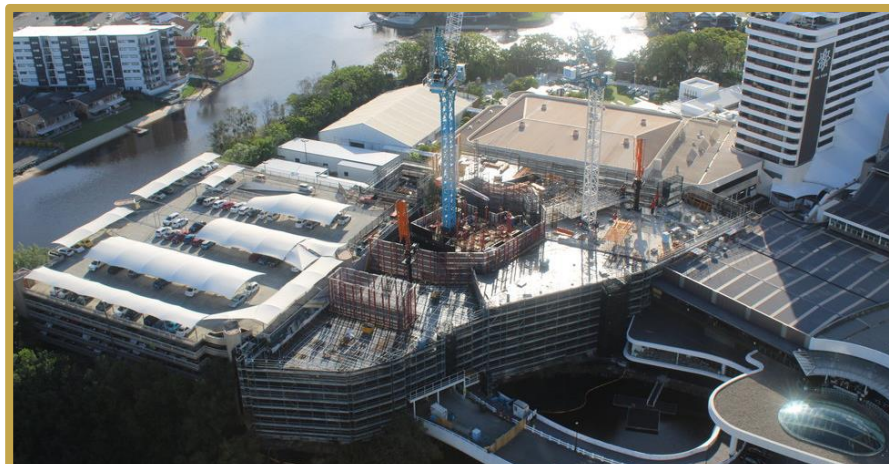
DORSETT HOTEL AND RESIDENCES (TOWER 1) FEBRUARY 2020
