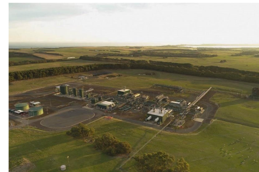
Minerva Gas Plant
